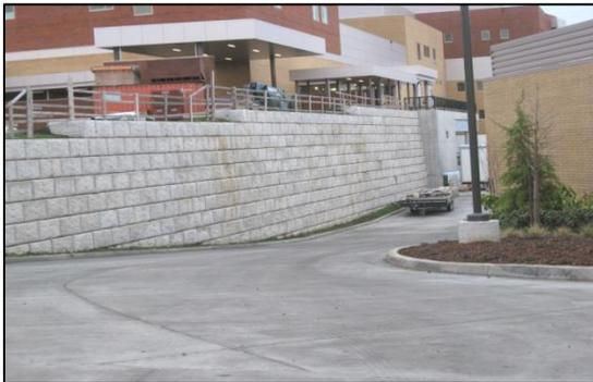
The project presented some challenges related to wall engineering. Wall heights of approximately 28 feet tall, seismic considerations, as well as significant loading from the actual hospital structure all needed to be well thought out. Time was critical and the start of building construction was dependent on the StoneTerra wall installation.
